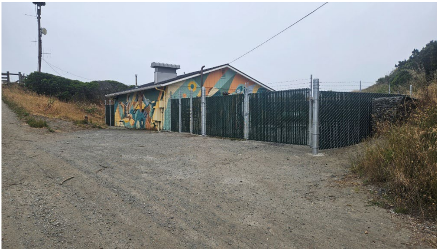
Completed Lift Station
