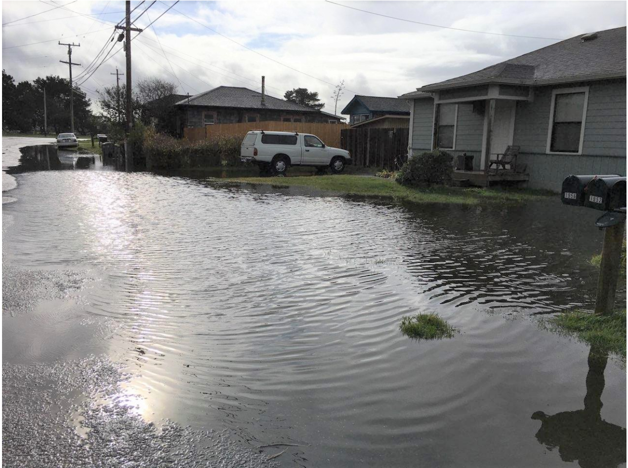
Figure 1. Common representation of flooding on Peninsula Drive due to Undersized, Failing Culverts and Drainage Channels. The proposed project will replace the failing culverts and implement bioswales.
