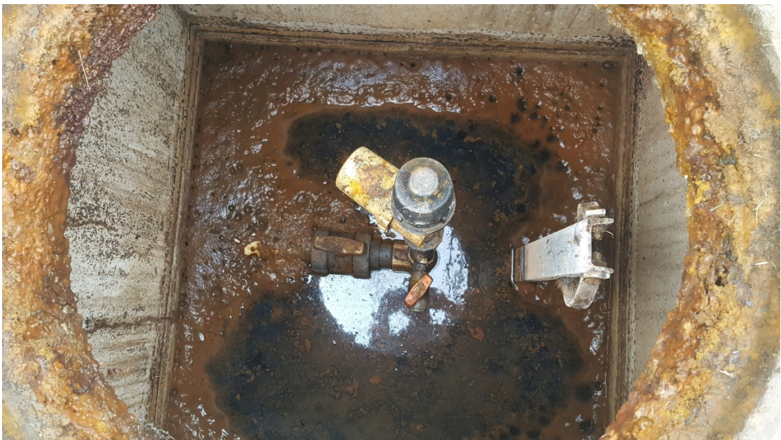
Figure 7. View of Air Release Valve (ARV) in a Vault.
