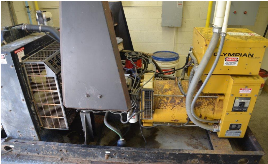
Figure 17. Standby Propane Powered Generator.
