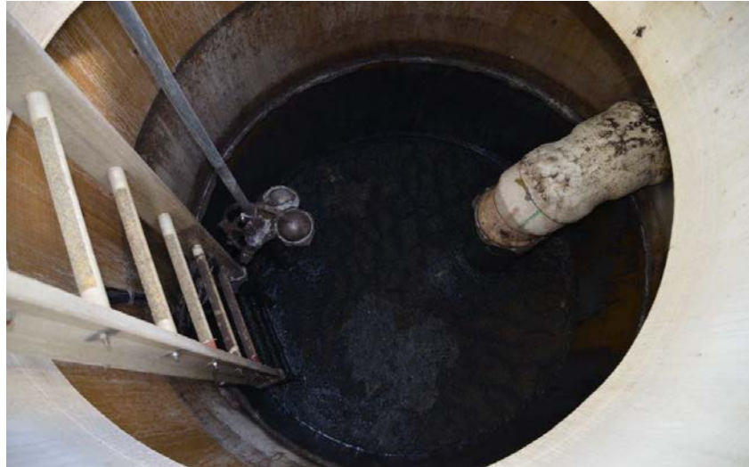
Figure 14. Original Wet Well Showing Influent Elbow to Reduce Odor Potential
