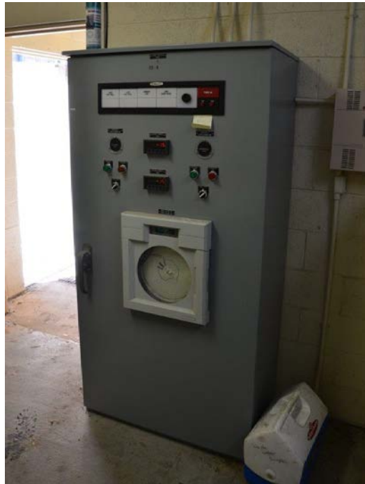
Figure 18. The Main Pump Station Control Panel
