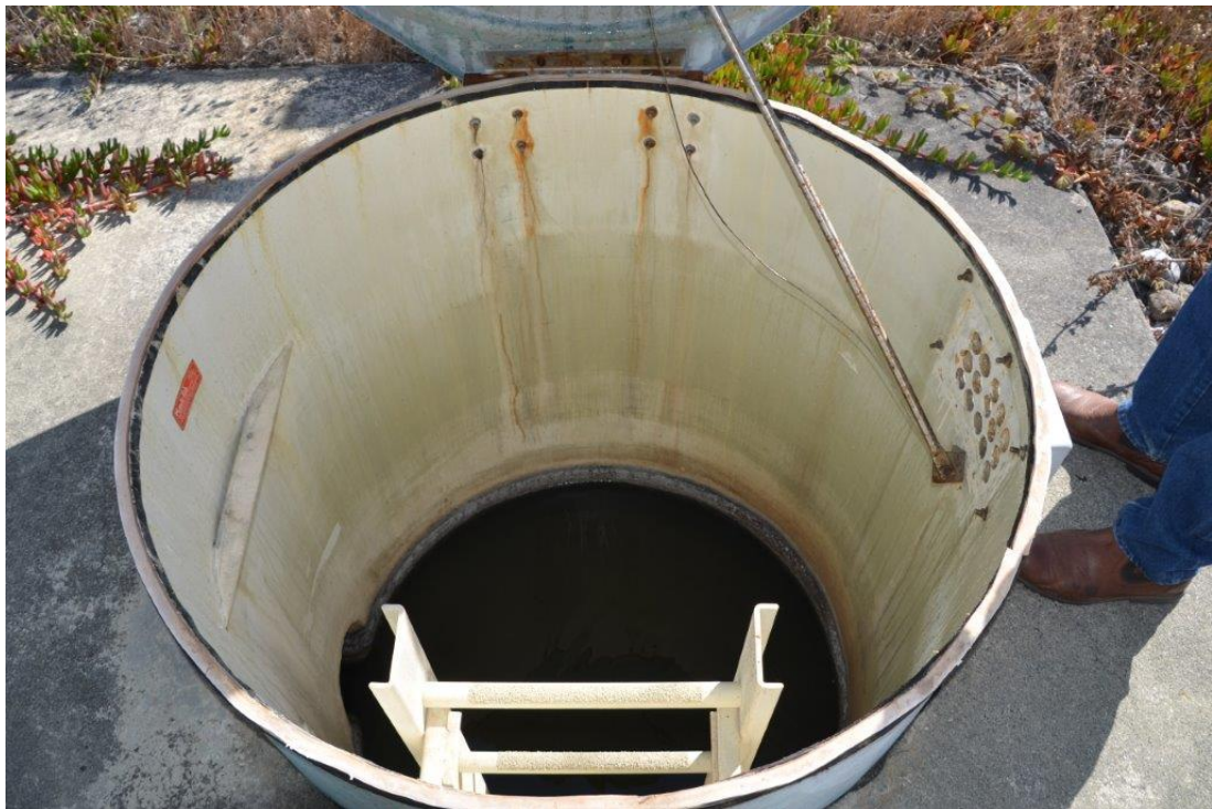
Figure 9. Grit Removal Vault
