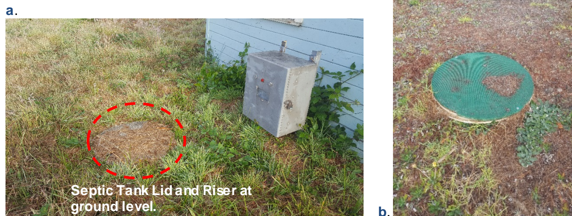
Figure 4. Examples of Septic Tank Risers at Ground Level
