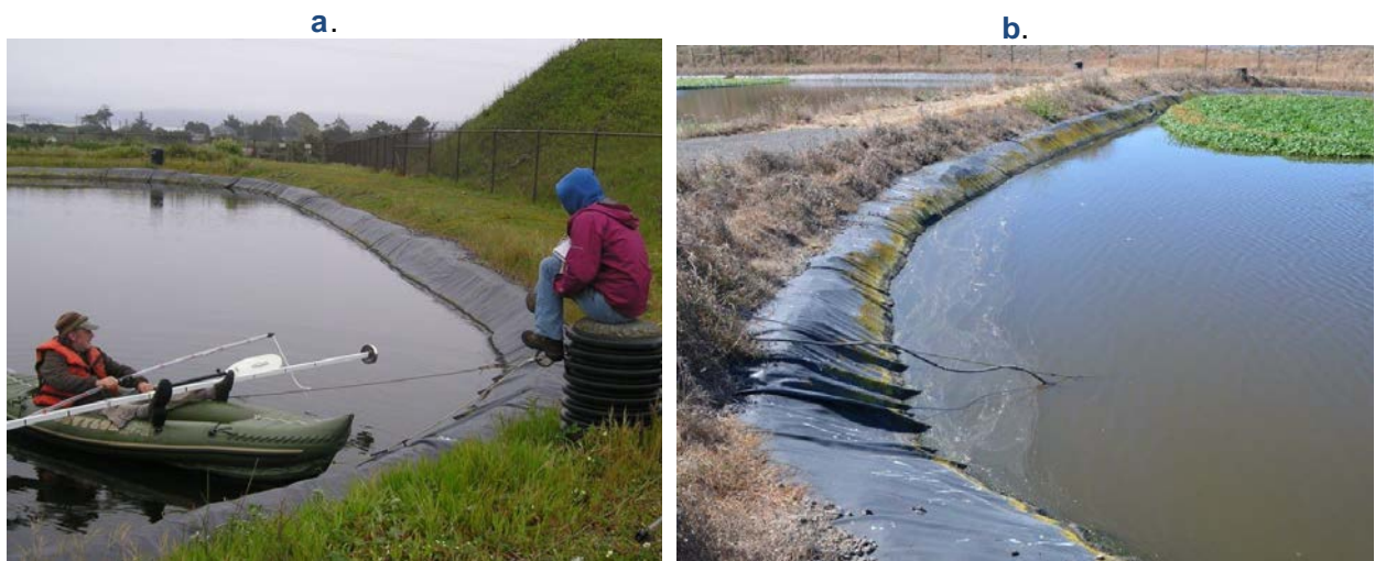
Figure 20. The Aerated Lagoon Impermeable Liners (a. 2006, b. 2018).
