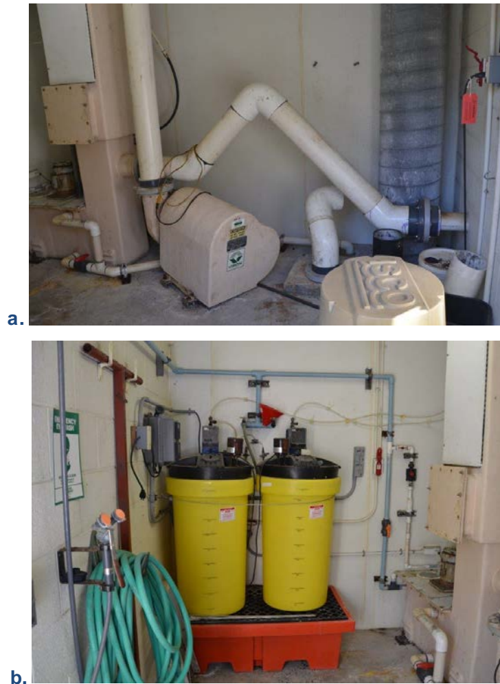
Figure 16. Unused Odor Control Equipment
