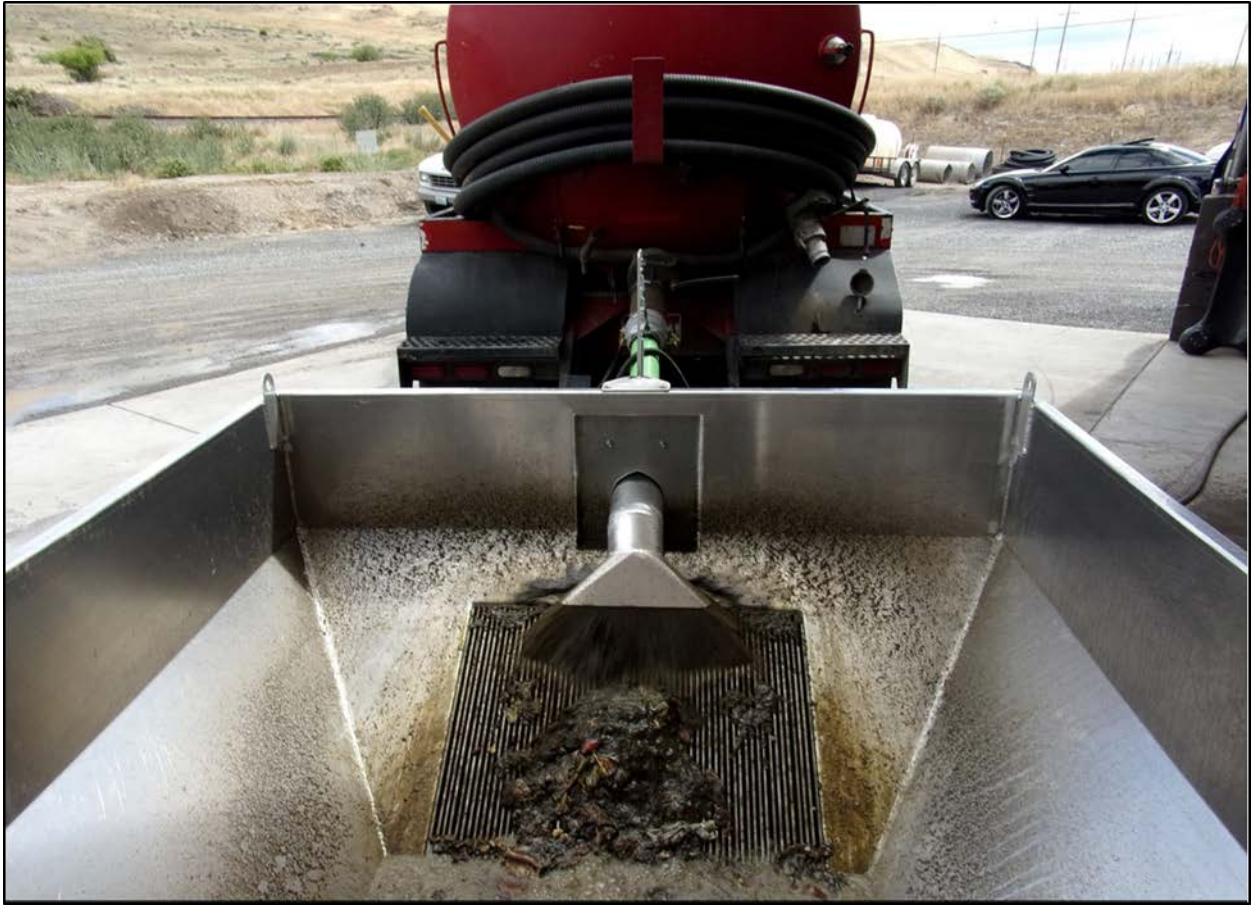
Figure 27: Septage being gravity fed into the ScreenCo Systems' MaxiScreen Product
