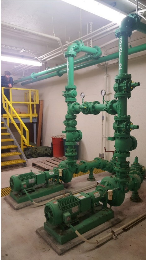
Figure 15. Two 5hp Pumps and Equipment within the Dry Well
