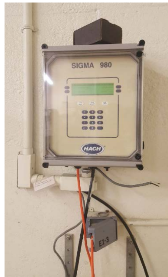
Figure 12. Hach Flow Meter and Data Recorder
