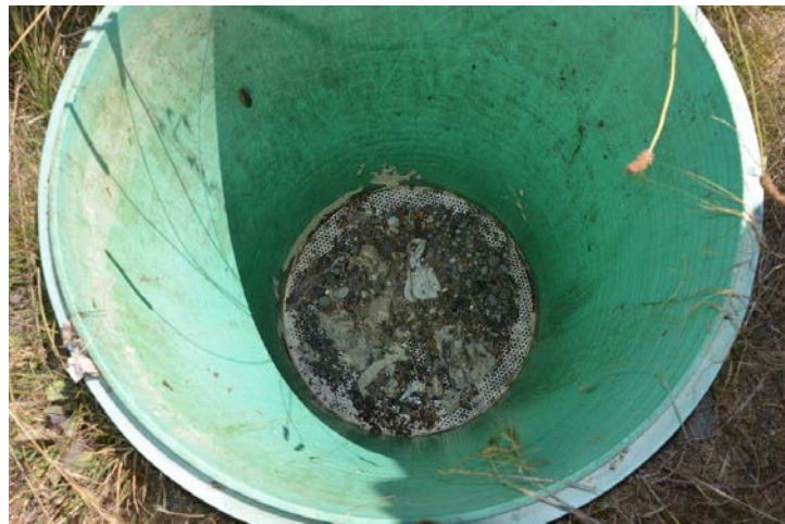
Figure 6. Septic Tank Riser with Screen at District Office
