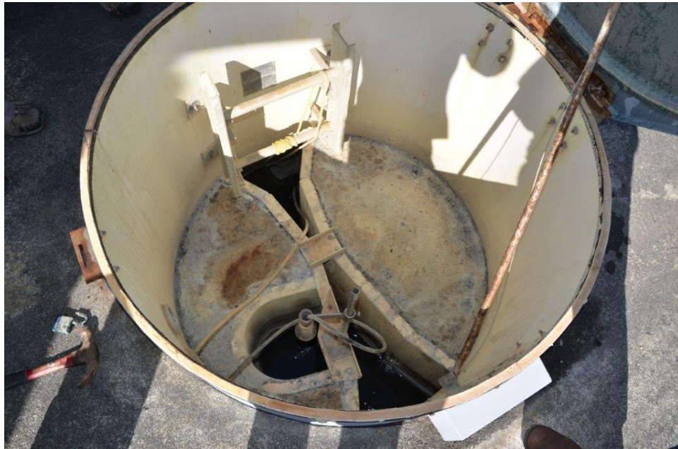
Figure 11. Influent Metering Vault with Parshall Flume
