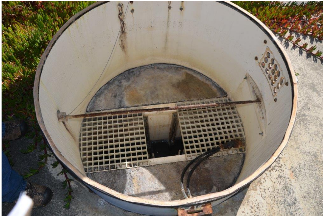
Figure 10. Grinder Vault. Note: Grinder Has Been Removed.
